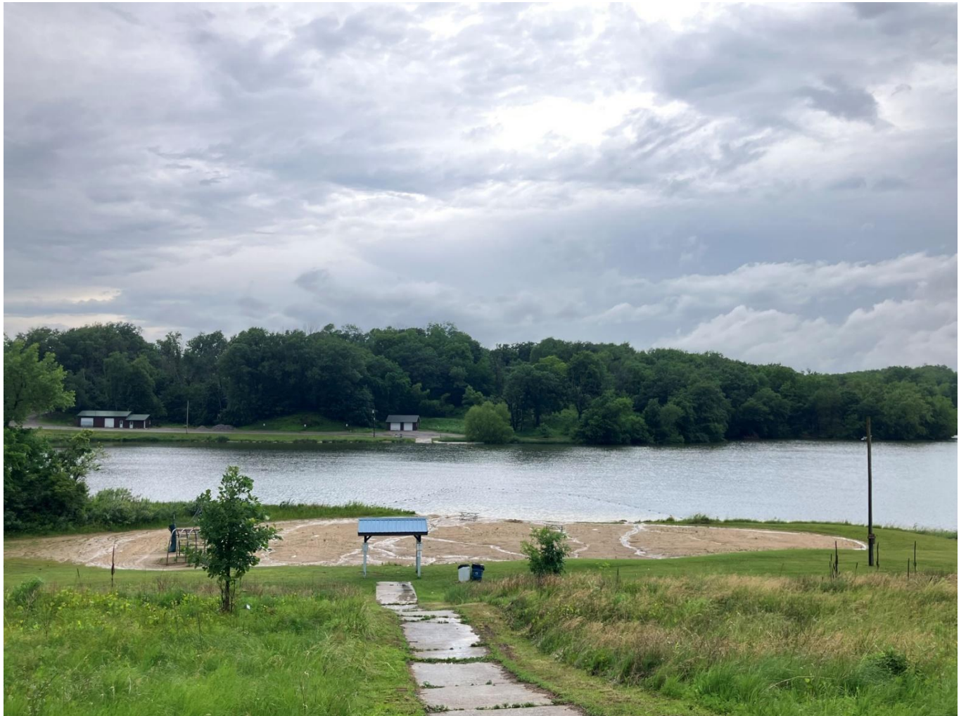
Figure 7. Photograph of the beach erosion at Hannen Lake caused by stormwater runoff.
