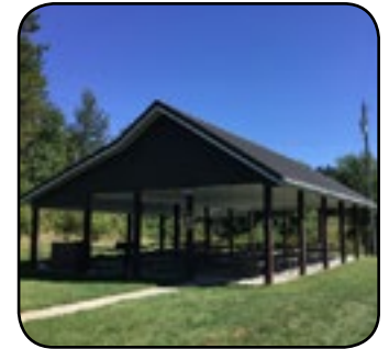
Renovated Hannen shelter
