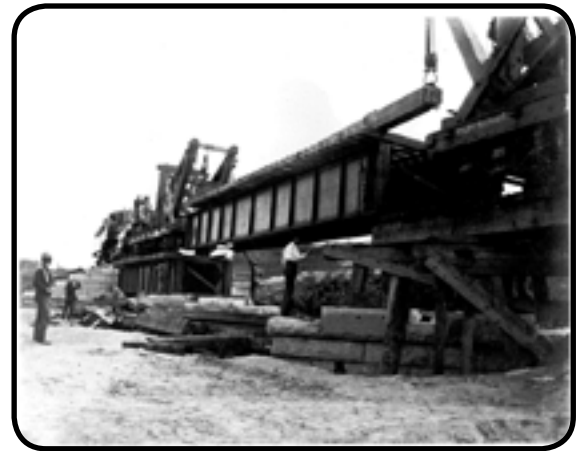
Old Creamery Nature Trail bridge construction
