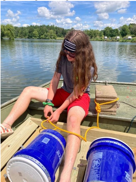
Figure 7: Will Cardo in Ranger Grubic's boat at Hannen Lake, attaching cinder blocks to the bottom of the docks with rope. The cinder blocks will keep the docks in place.
