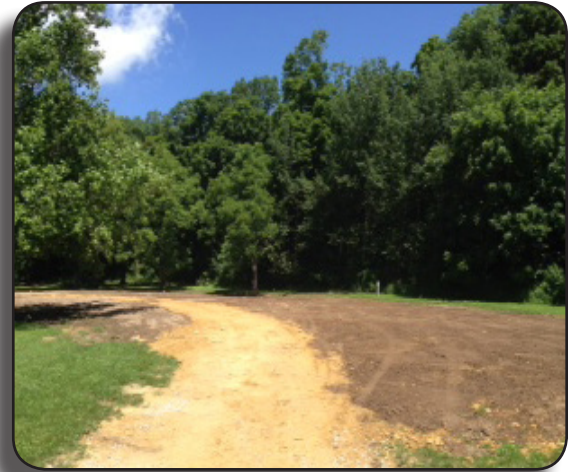
Looking East, several campsites at Wildcat Bluff Park were raised four feet to bring the sites to a level grade. Top soil was replaced using fill from the playground addition.
