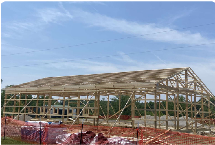
Figure 3: New Hannen Lake Park shop construction.
