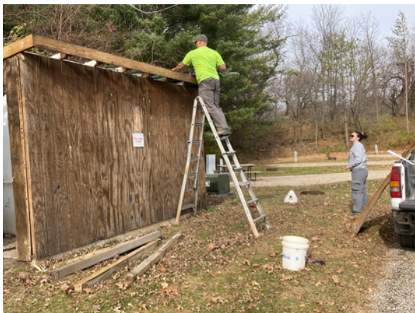
Figure 8: Rangers removing old pit toilets.
